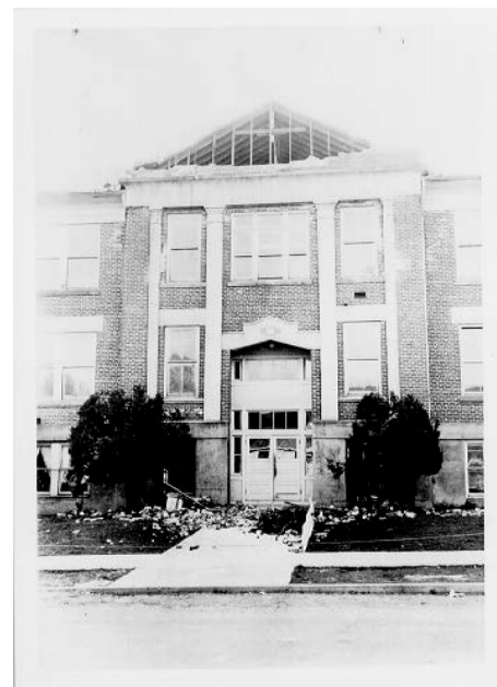
1949 earthquake, Washington State. Gables on a number of unreinforced masonry school buildings collapsed; fatalities recorded.
